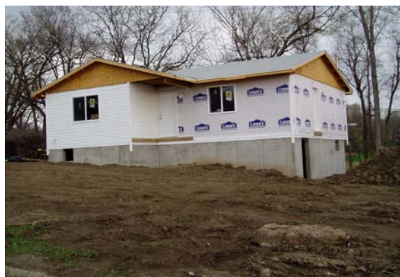
Home now under construction at 2516 Rose Lane
