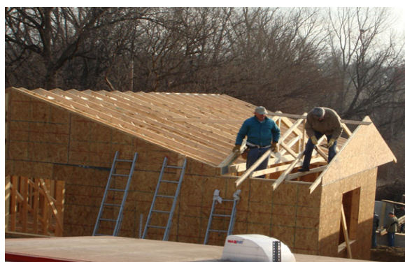
Construction Chair Jim Arbuckle helps a volunteer put up trusses
